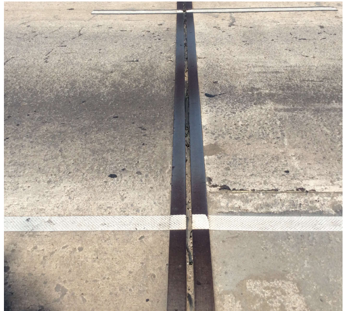
PHOTO 2 Description Compression seals are deteriorated and torn.
