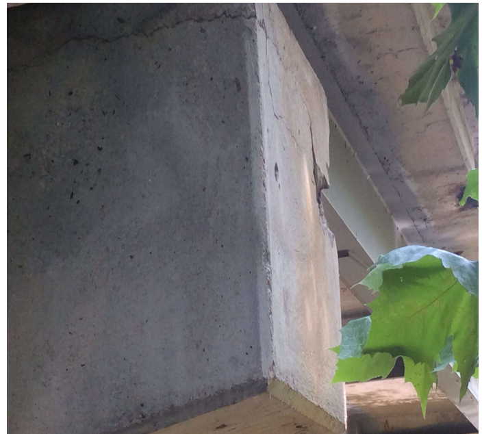
PHOTO 2 Description Bent 2 has a 16" delaminated area in the Rt end of cap.
