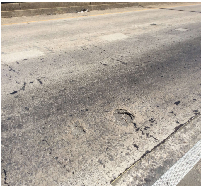
PHOTO 1 Description The driving surface of the deck has spalling with delaminated areas in the right lane and gutter.
