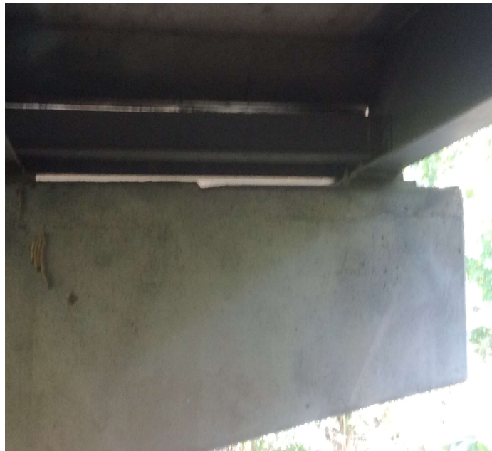
PHOTO 1 Description The Rt side of Bent 2 cap has horizontal cracking approximately 6" below the top of the cap on the Span 1 and Span 2 sides.
