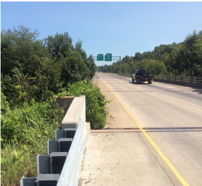
PHOTO 1 Description Vegetation beginning to grow into the edge of the shoulders on the bridge railing.
