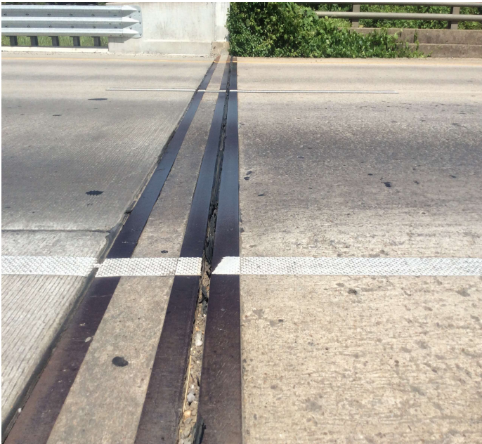
PHOTO 1 Description Compression seals are deteriorated and torn.
